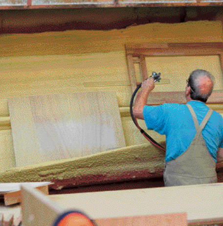
Top left: Evernew's production manager, Darren French, displays the 70mm Oregon roof beams checked into the walls. Top right and above: The Evernew team builds up to 3.5 vans a week.
